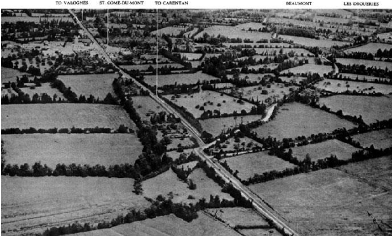
Aerial View of Dead Man's Corner
